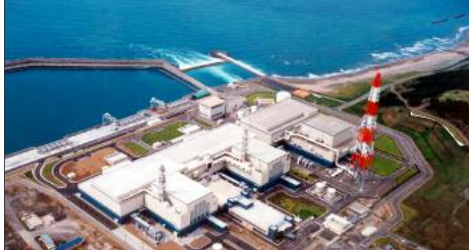
Three of the seven reactors at Kashiwazaki-Kariwa, the world's largest nuclear power station.
