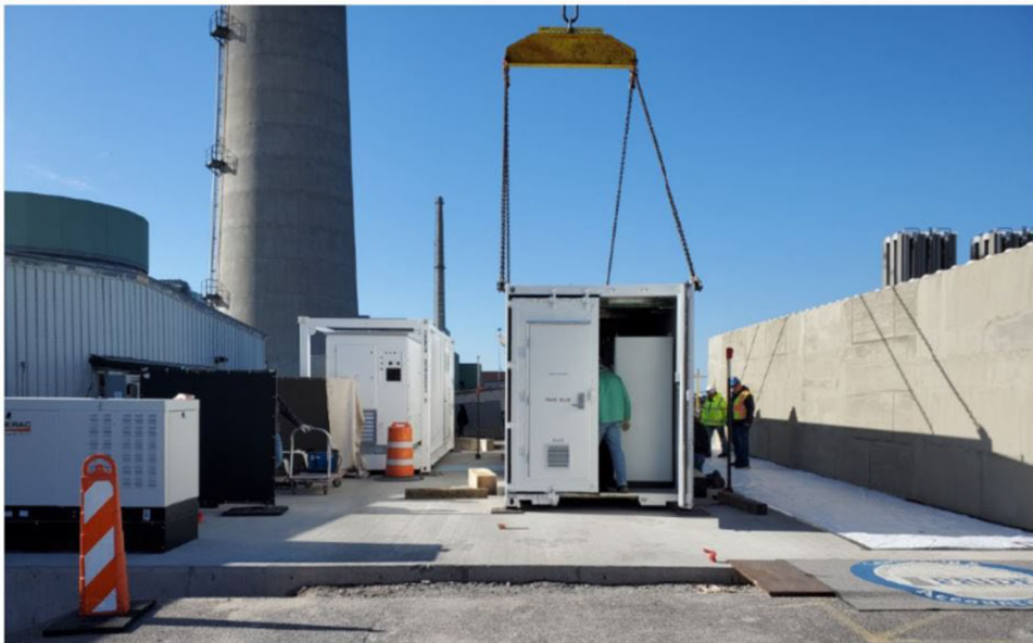
Graphic 1 - Installation - Rigging Electrolyzer into Place
