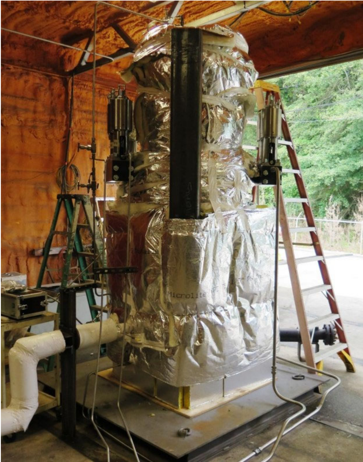
Figure 4 – New SMA MSIV Actuator Hot Functional Testing During Fabrication
