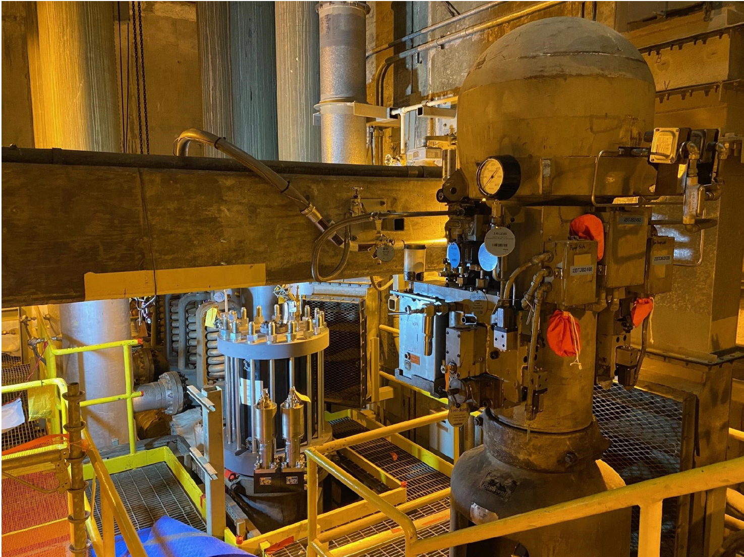
Figure 2 – MSIV Actuator Comparison – Legacy in Foreground vs. New SMA Actuator in Background
