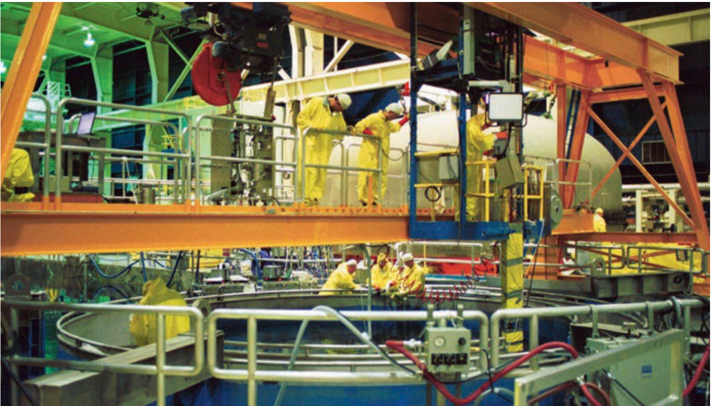
Crew inspecting reactor vessel internal components, part of an extensive maintenance program.
