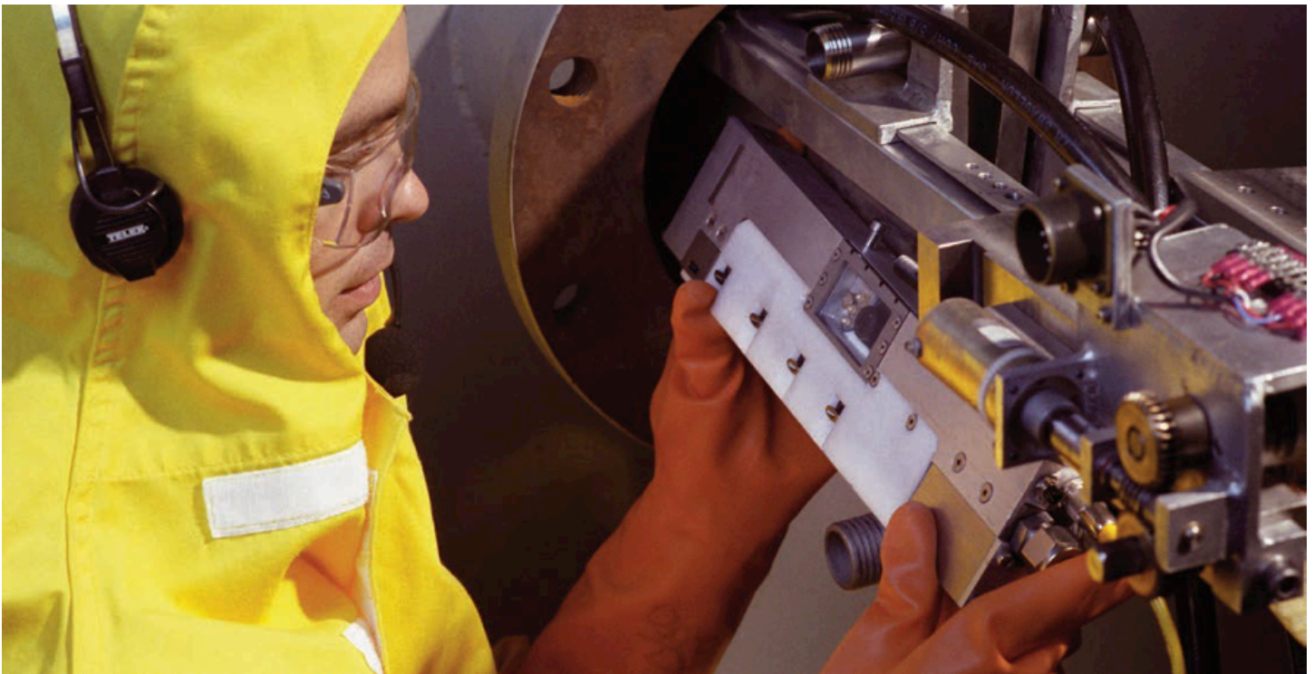
A nuclear technician training on the proper installation of steam generator water lancing equipment used for cleaning.
