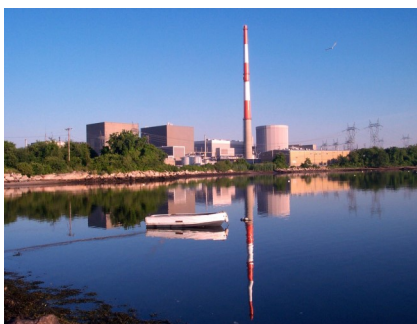
Millstone Power Station
