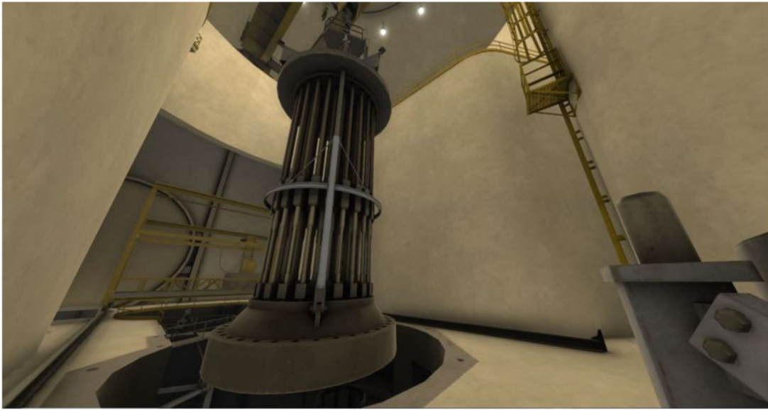
Figure 3: View from the floor while lifting a reactor head
