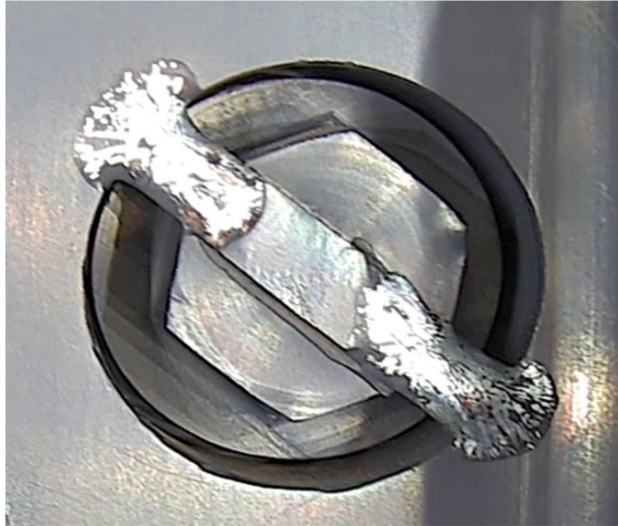
Figure 2 – Typical External Hex Clevis Insert Bolt with Locking Bar and Excessive Weld Material
