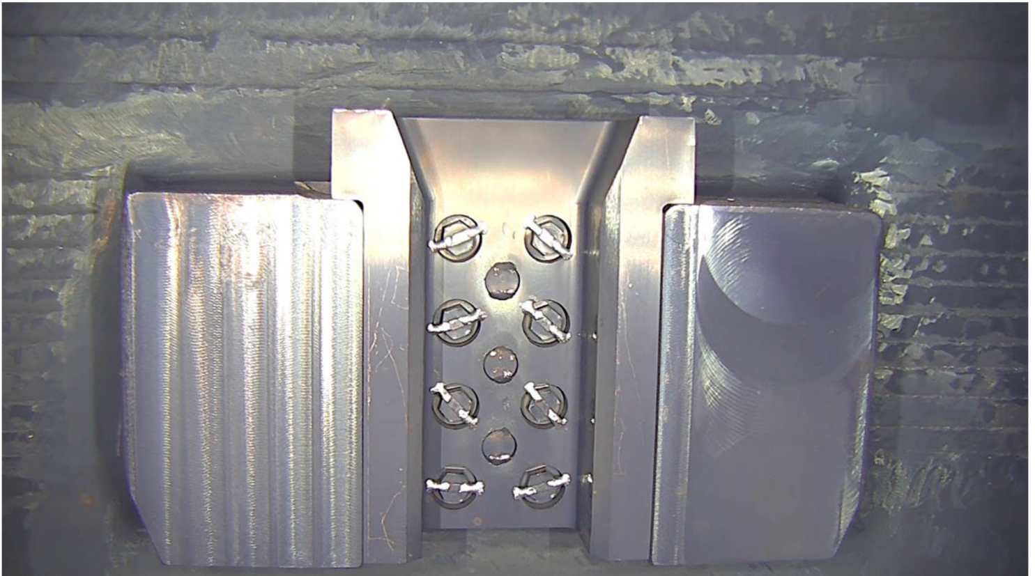
Figure 1 - Lower Radial Support Clevis and Insert
